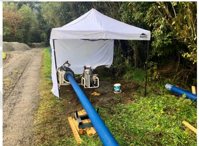
Fox Glacier Water Treatment Plant renewal work
